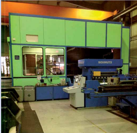
Production / Line cabin / Cut-to-length-line
